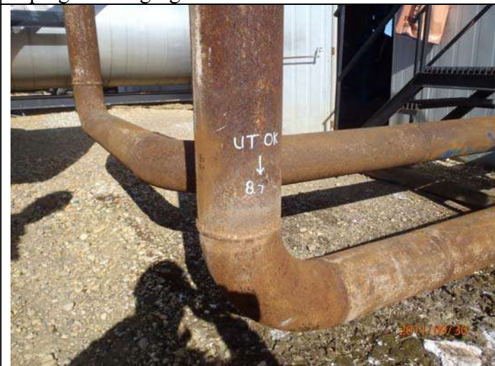
Lowest reading 8.7 mm on Elbow.
