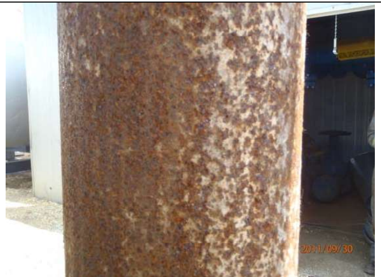
Piping showing light corrosion – pitted surface
