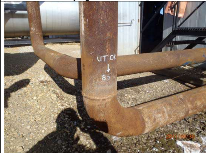
Piping showing light corrosion
