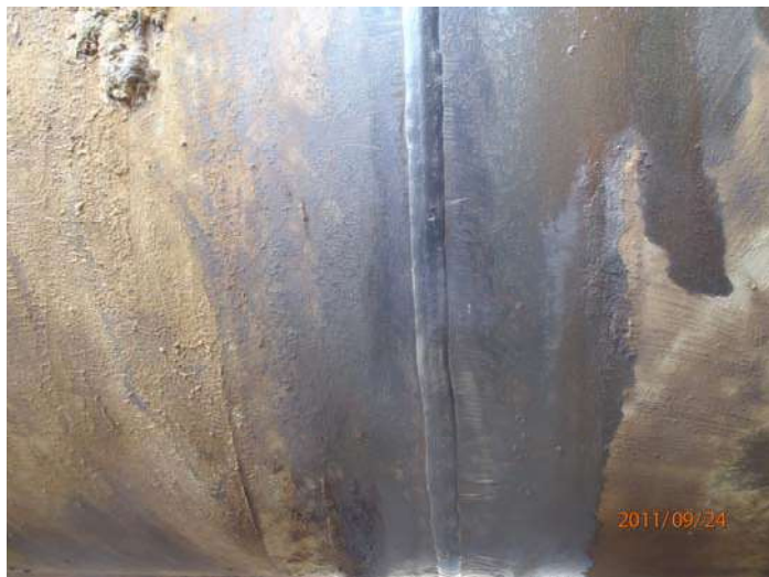
Welds were Power Brushed to clean
