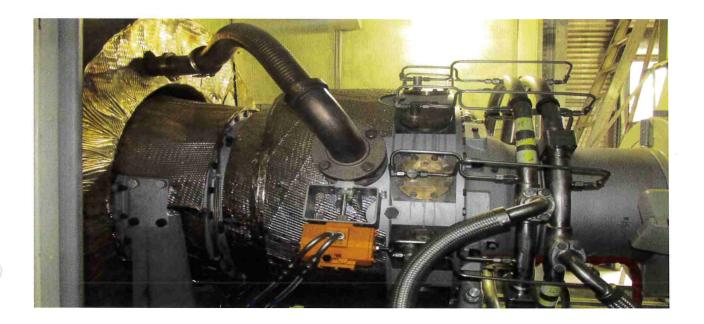
A: The turbine engine air inlet system components (air filters, ducting, and silencer).
