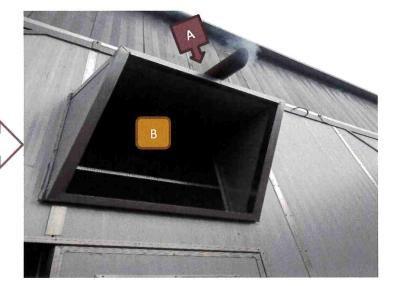
Turbine exhaust system, pressure loss should not exceed 6 inches of water; additional back pressure results in a decrease of available horsepower.
