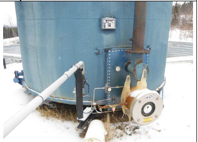
Tank support // Lower shell // Manway
