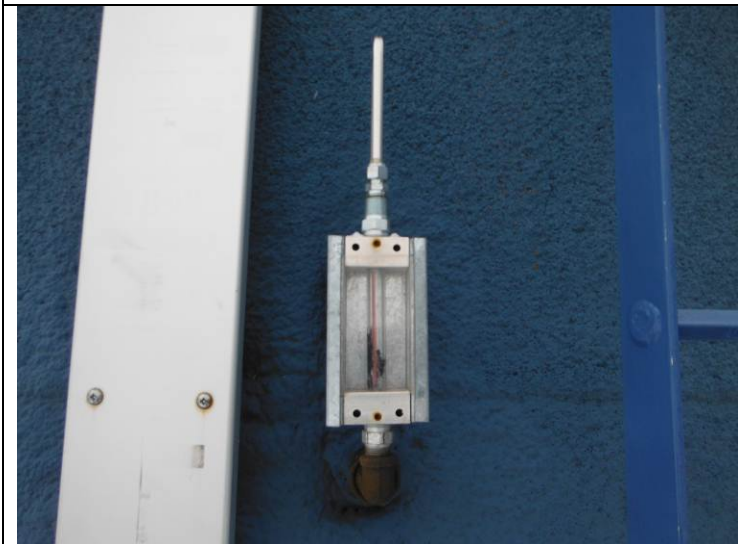
Interstitial level gauge
