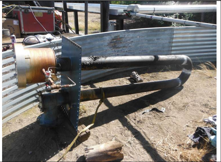
Fire tube - no cracking detected
