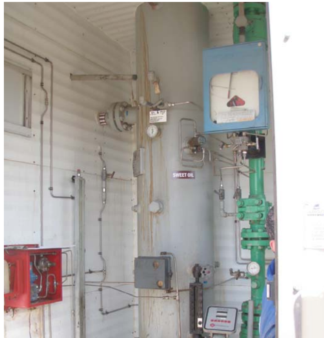
02-A0404024 Overview Inside
