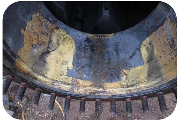
A2710237_Manway nozzle in good shape_10Oct2012
