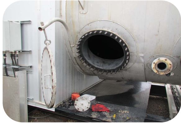
A2710237_South West manway_10Oct2012
