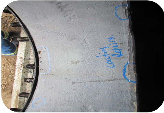
A2710237_Coating repairs on the manway nozzle_10Oct2012
