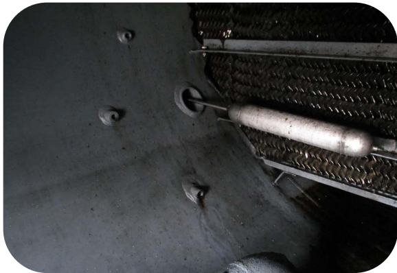
A2710237_Level float gauge_10Oct2012
