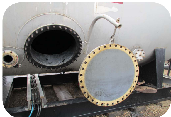
A2710237_South East manway and cover_10Oct2012
