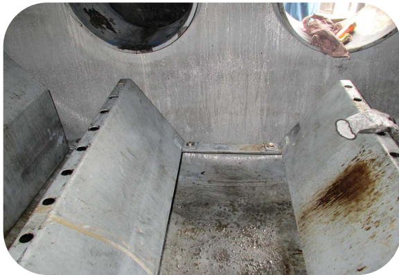
A2710237_Supports intact and secure_10Oct2012
