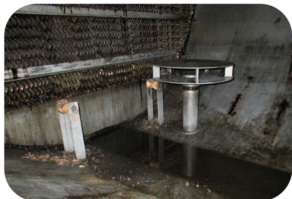
A2710237_Inlet deflector_10Oct2012
