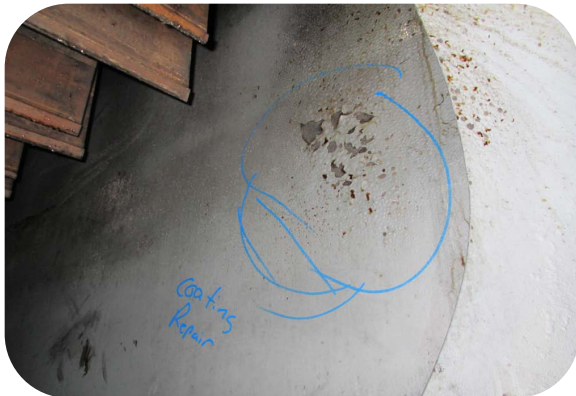
A2710237_Coating repair on weir plate_10Oct2012
