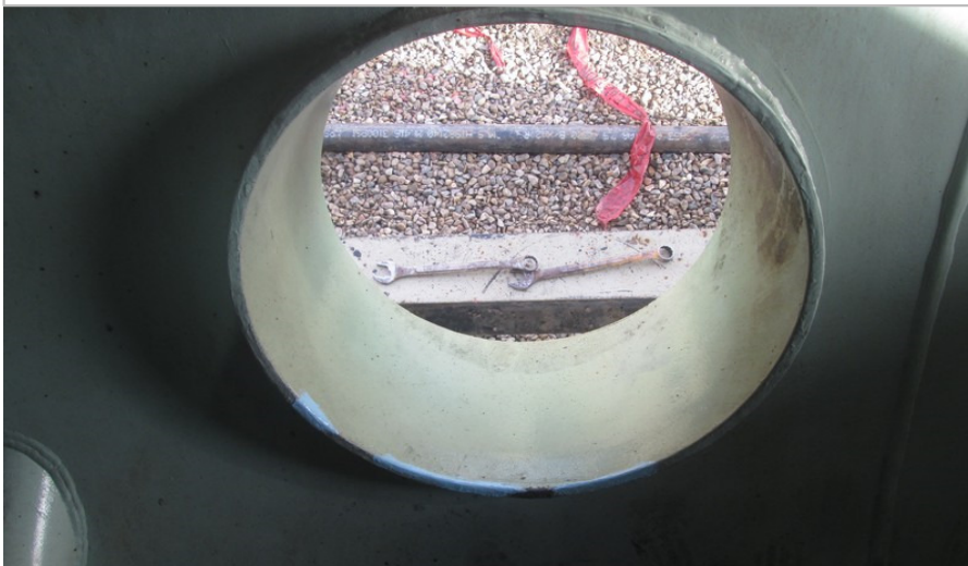
Coating holidays at 6:00 in shell and on manway cleaned and Devco 142 applied.
