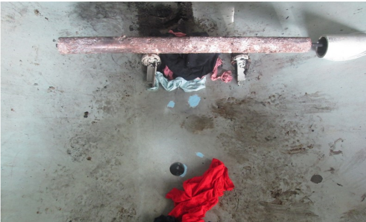
Coating holidays at 6:00 in shell and on manway cleaned and Devco 142 applied.
