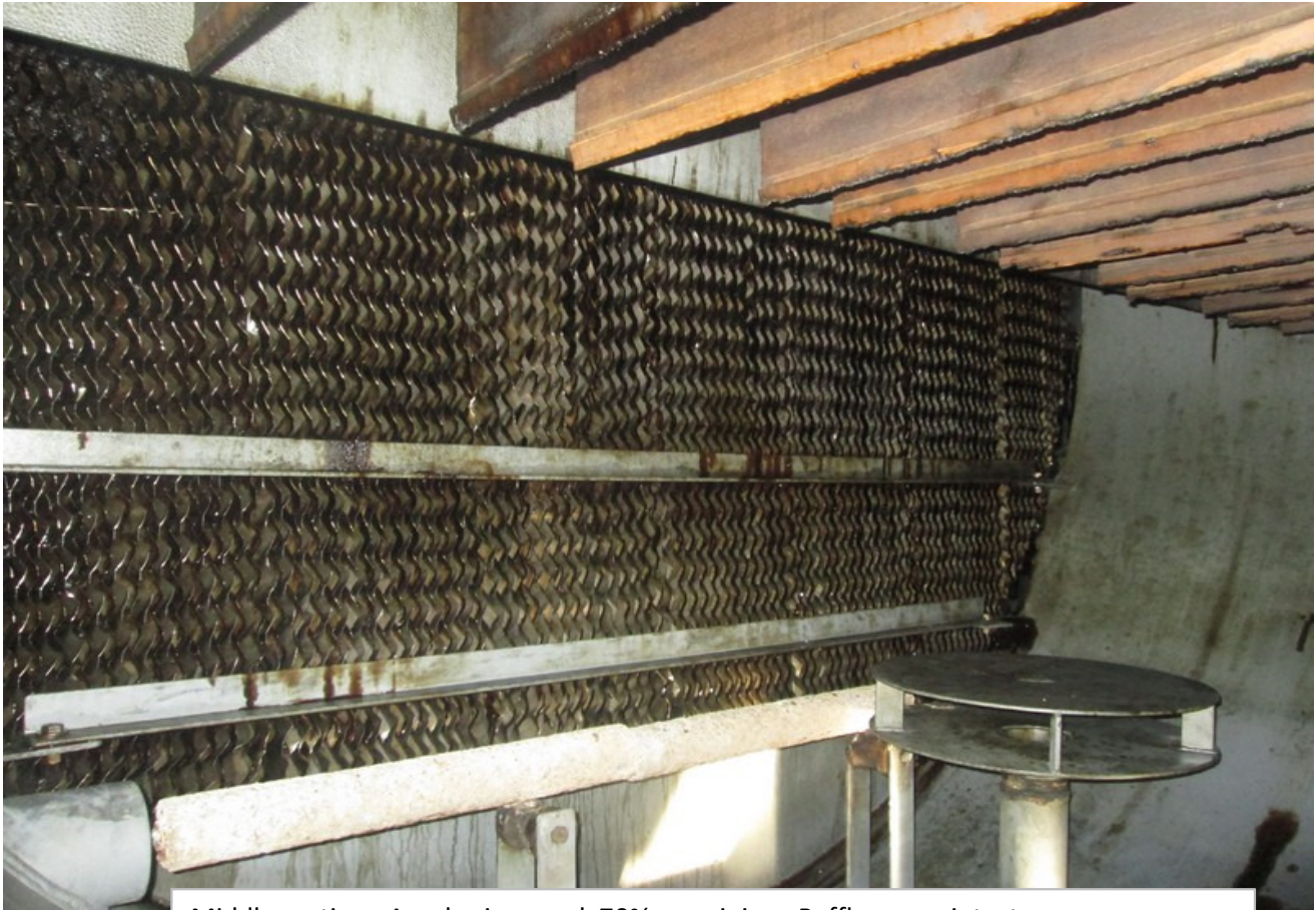
Middle section. Anodes in vessel, 70% remaining. Baffle group intact.
