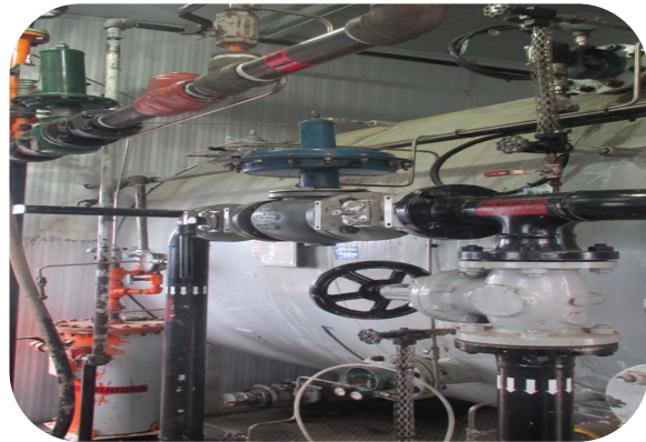
A2710237_North shell inside building_9Sept2014
