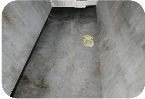
A2710237_East bottom shell coating intact_9Sept2014
