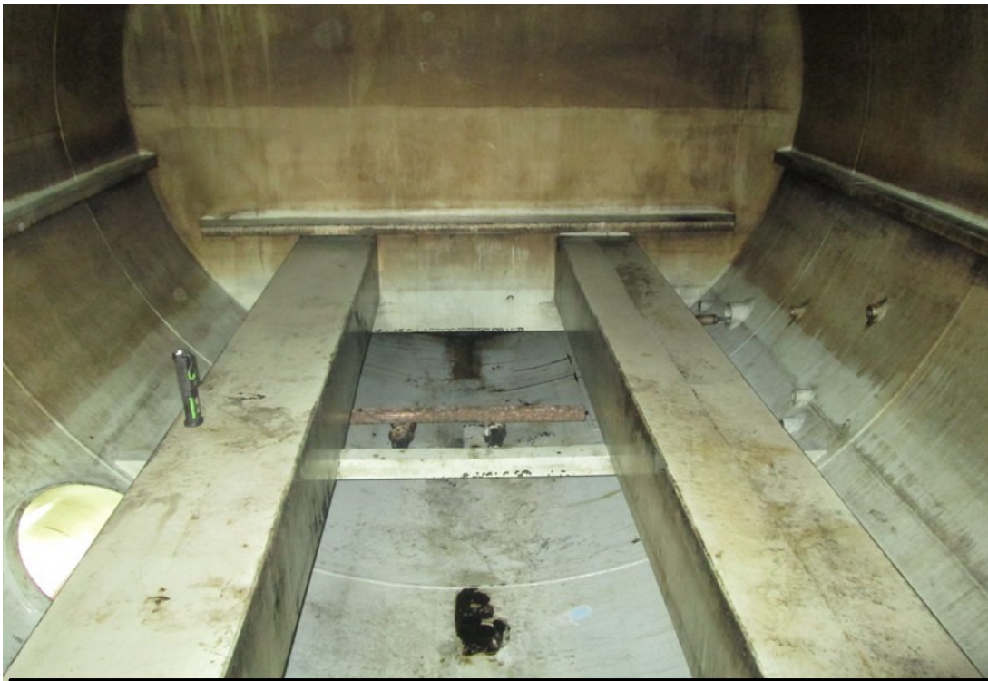
Minor holidays at 6:00 position in shell were cleaned and Devco 142 applied.
