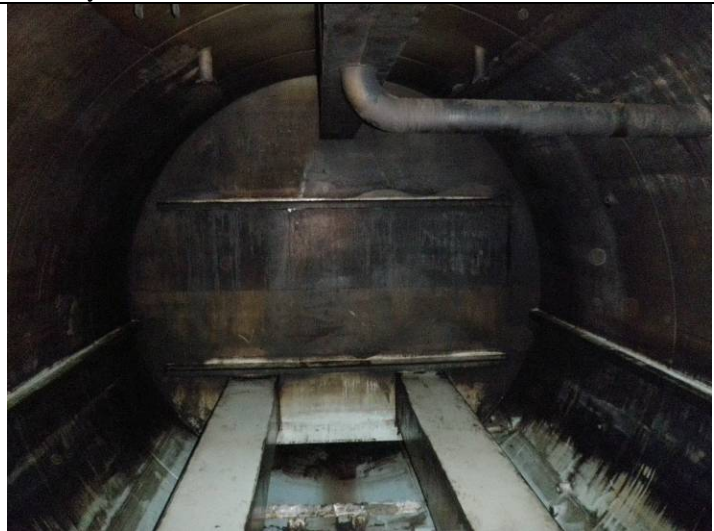
Overview of rear shell, piping and weir
