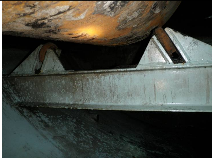
Fire tube support & rollers
