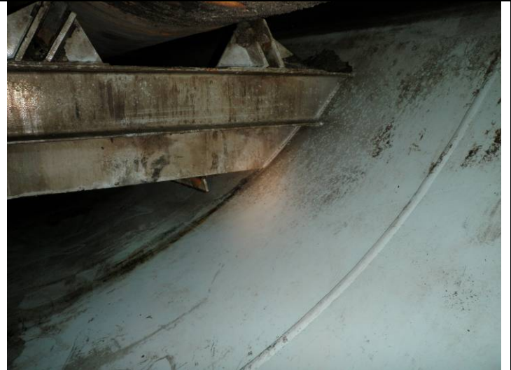
Fire tube support & rollers
