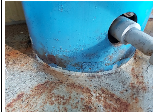
Base welded to floor
