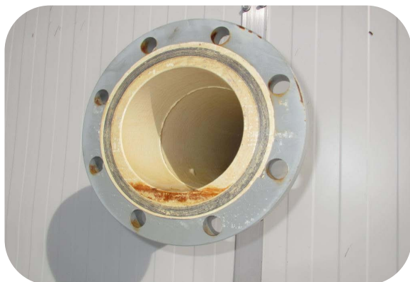
C38332_South End 6" Inlet nozzle coating and gasket surface intact_18March2013
