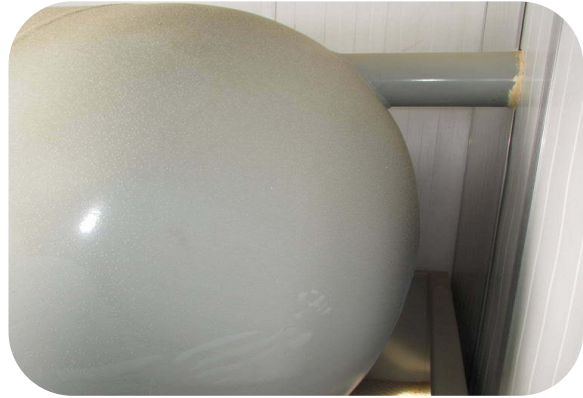
C38332_North end Head and 6" Inlet Nozzle_18March2013
