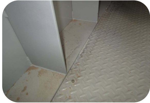
C38332_Saddles welded securely to floor and shell_18March2013
