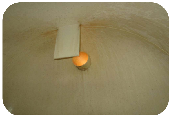
C38332_North End 6" Inlet Nozzle and deflector plate intact_18March2013
