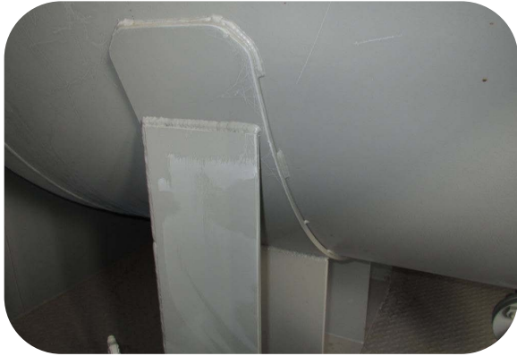
C38332_Saddles welded securely to floor and shell_18March2013
