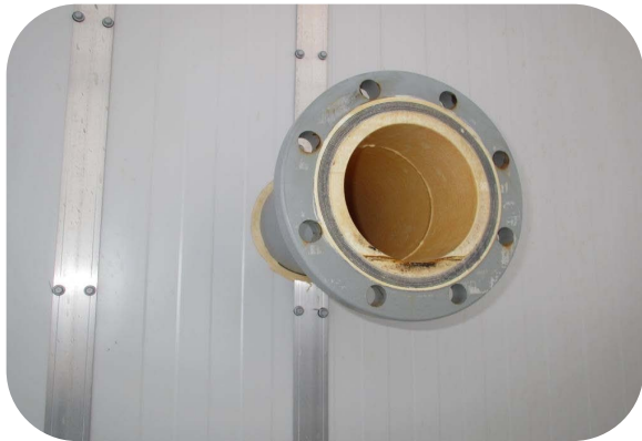
C38332_North End 6" Inlet nozzle coating and gasket surface intact_18March2013
