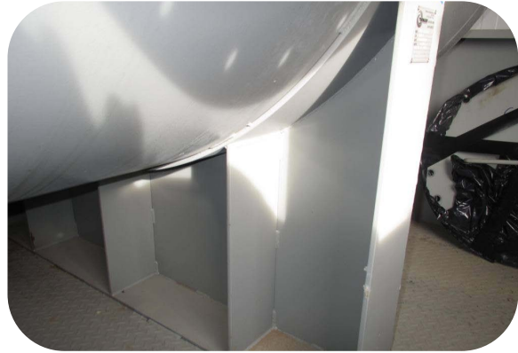
C38332_Saddles welded securely to floor and shell_18March2013
