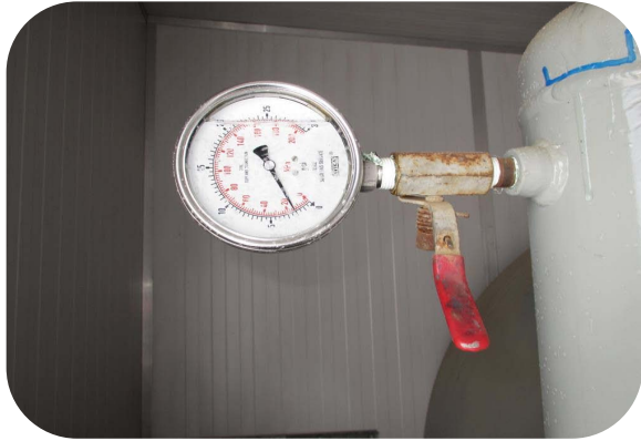
C38332_Pressure gauge not working properly _18March2013
