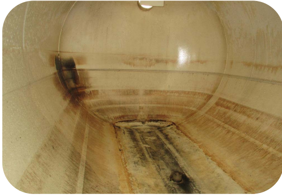
C38332_Internal view of south shell , head and internal coating intact_ 18March2013
