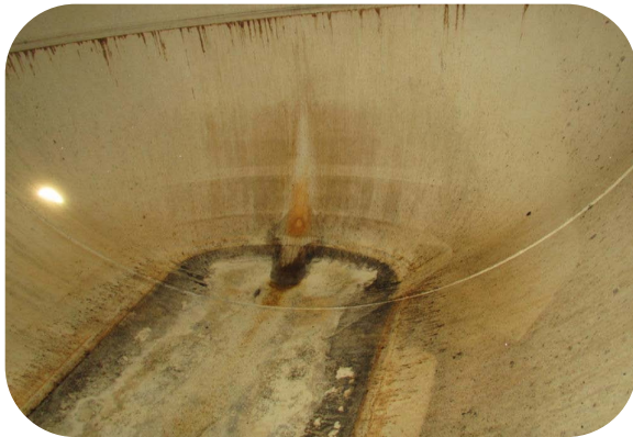
C38332_North End shell and head coating intact_18March2013
