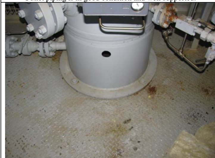
Skirt is in good condition with anchor bolts tight.
