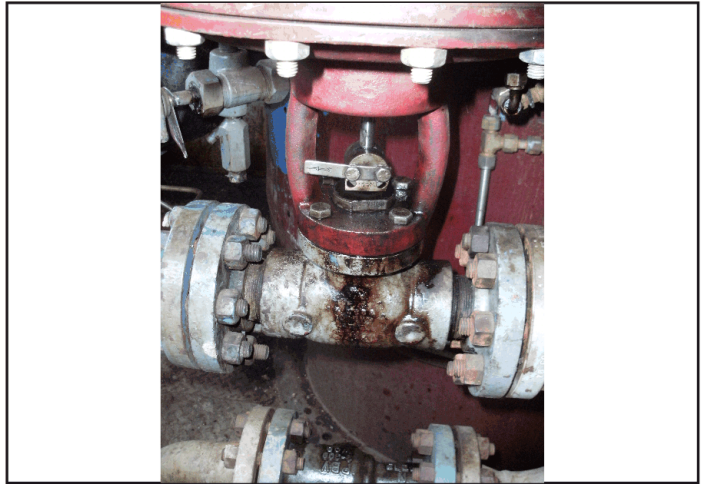
SEEPAGE ON ACTUATOR VALVE
