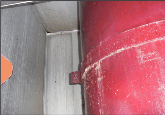
PAINT FLAKING AND RUSTING ON SHELL
