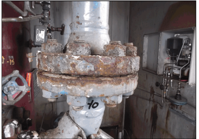
PIPING CORROSION
