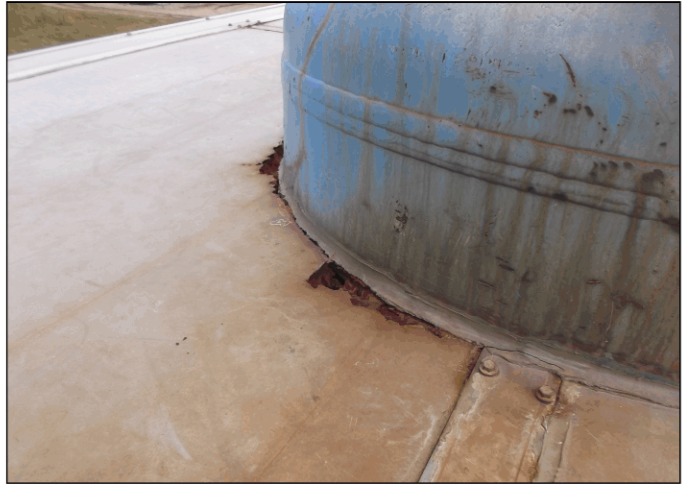
ROOF CORROSION
