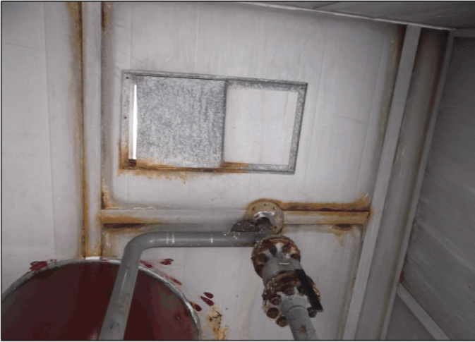
ROOF CORROSION
