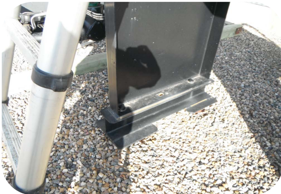
A2664161_Vessel supported on saddles_14March2012
