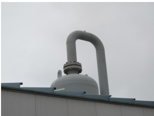
Top head above roof
