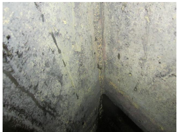
Baffle plate to shell weld
