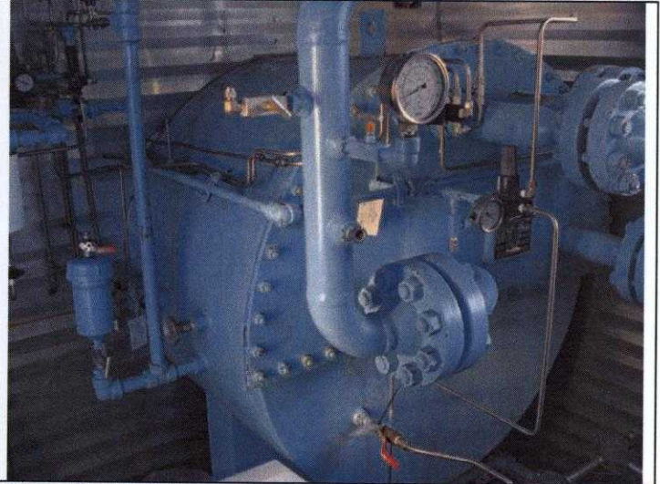
View of the insulation.
