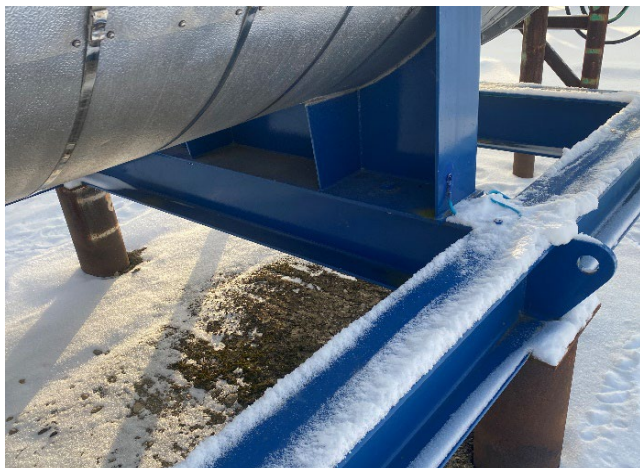
Picture 5: Saddle and directly grounded
