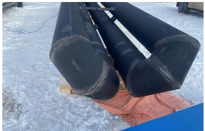
Picture 2: Miter Welds
