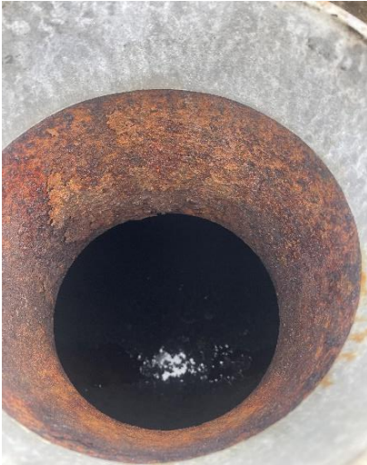
EXPANSION TANK THIEF HATCH NOZZLE NECK
