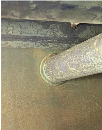
TYPICAL PROCESS COIL SUPPORT TO SHELL WELD
