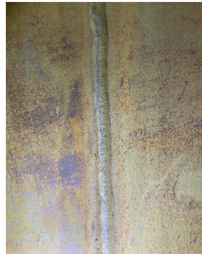
TYPICAL WELD SEAM CONDITION
