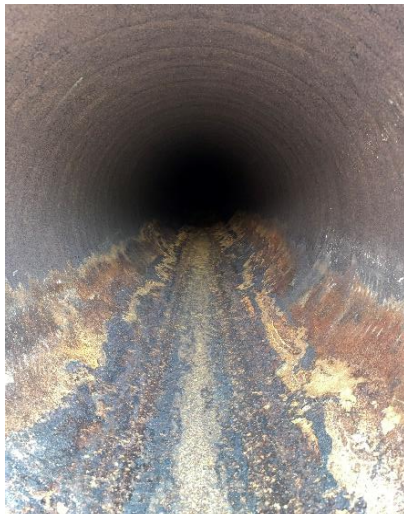
STACK SIDE INTERNAL OVERVIEW
