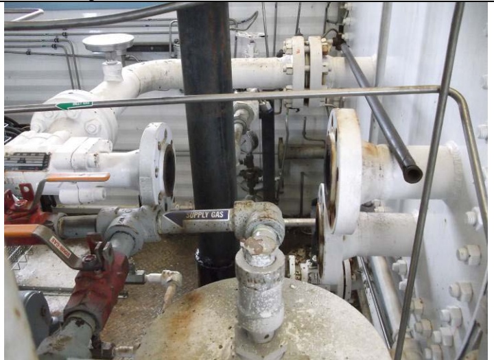
Piping disconnected
