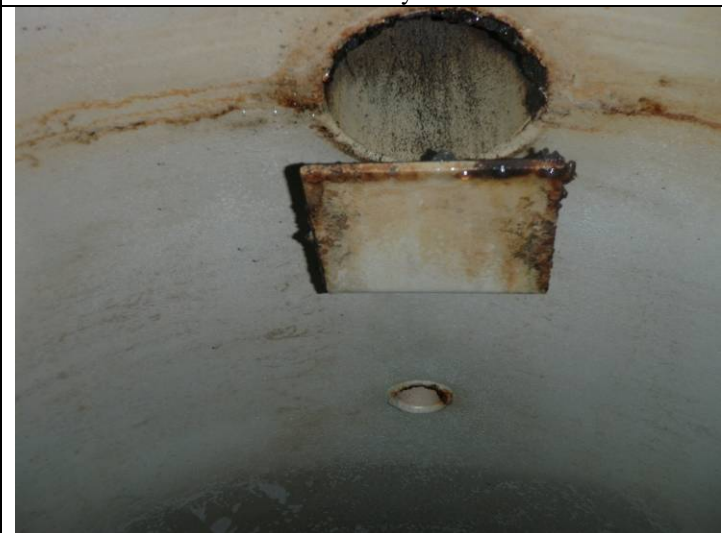
Inlet nozzle and deflector plating
