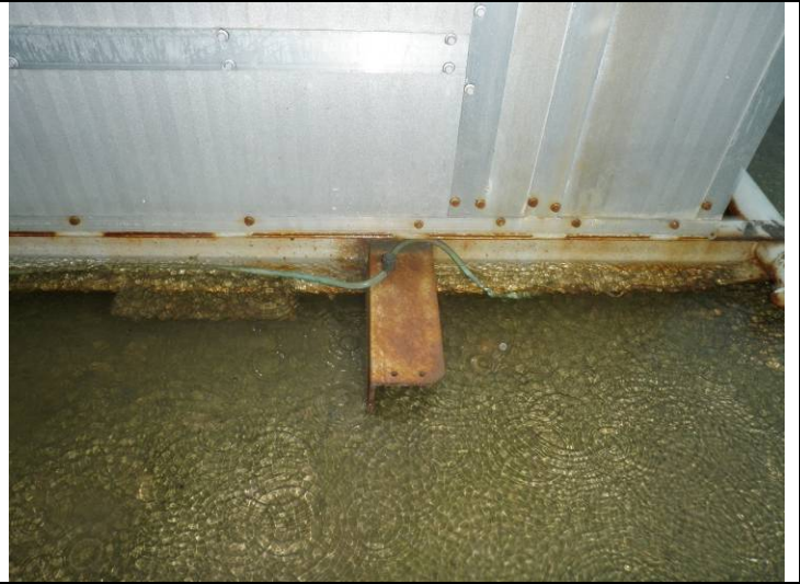
Ground wire attached
