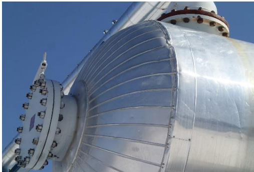
Figure 3: Overview outside building
