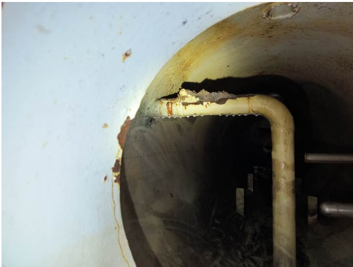
Picture 4: East head / inlet deflector plate
