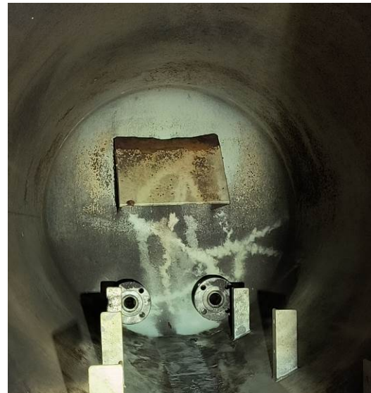
Picture 4: East head / inlet deflector plate
