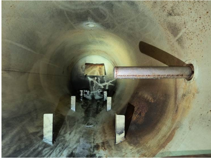
Picture 5: Coating burned for catadyne heater
