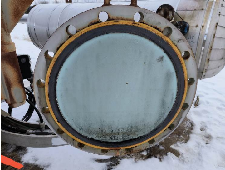
Picture 2: Manway / Coating damage
