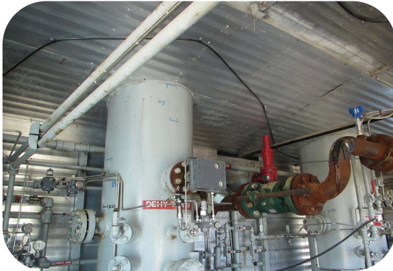
A0437520_Middle section roof to shell interface view_29August2013
