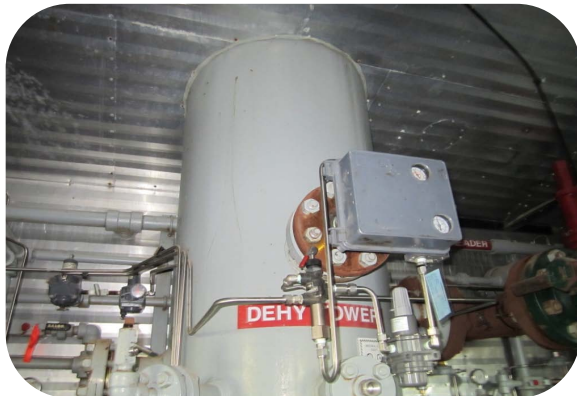
A0437520_Shell to roof interface_30Mar2012
