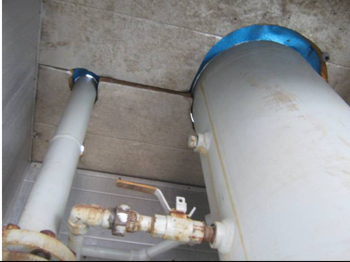
Roof closure not sealed – egress of moisture
