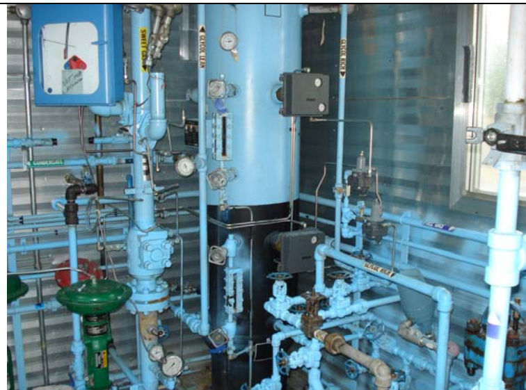
View of shell below roof.
