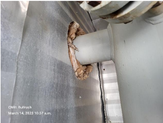
Inlet piping overview
