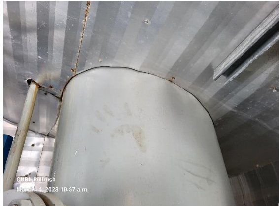
Roof seal overview
