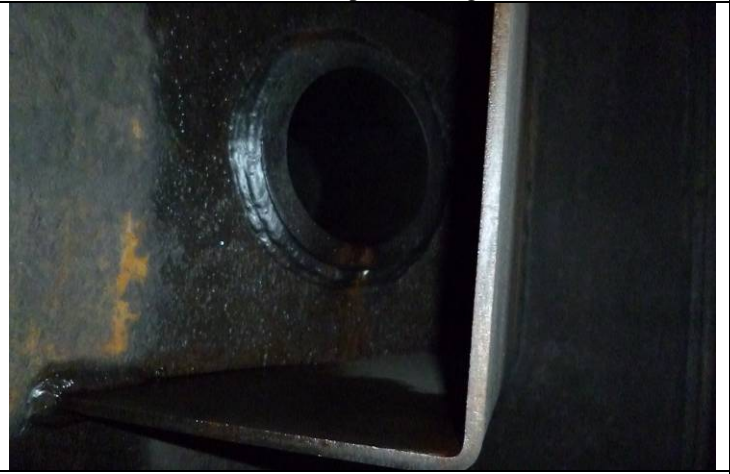
Inlet nozzle and deflector
