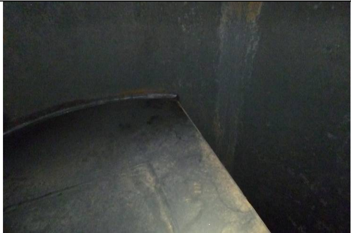
Cover attachment weld to shell
