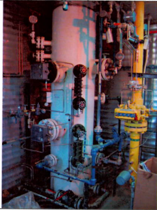
Inside Overview photo
