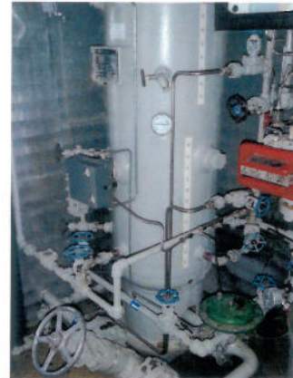
Vessel Lower Shell & Bottom Head View
