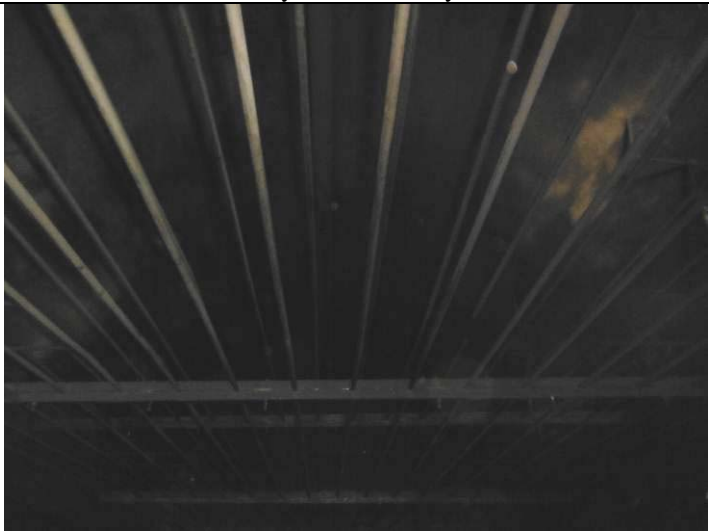
Overview Dry side grid
