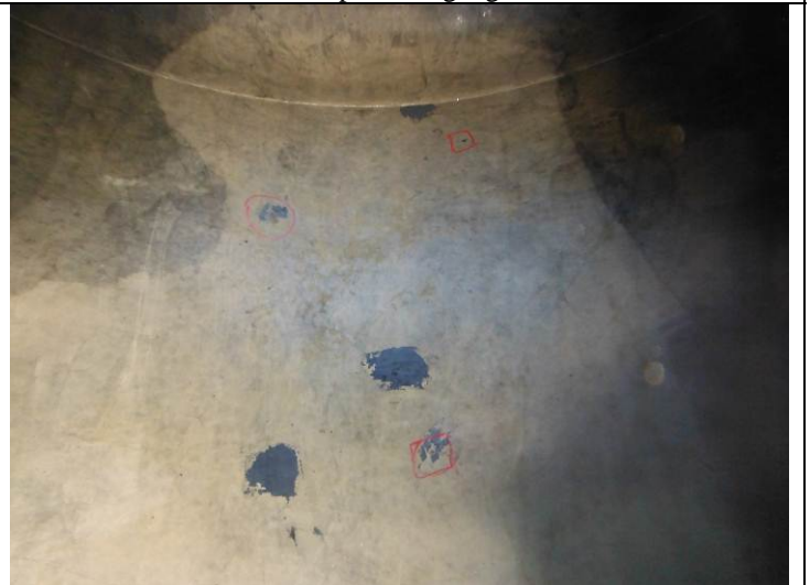
Bottom shell – several coating chips
