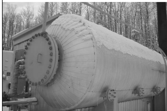
vessel overview of manway
