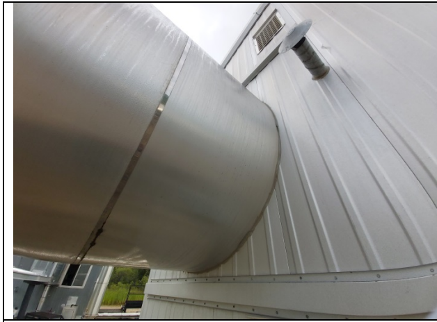
Wall to shell sealed
