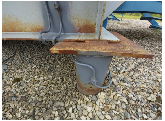
Ground cable attached
