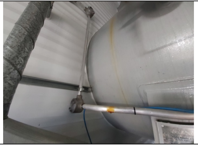
Wall to shell sealed
