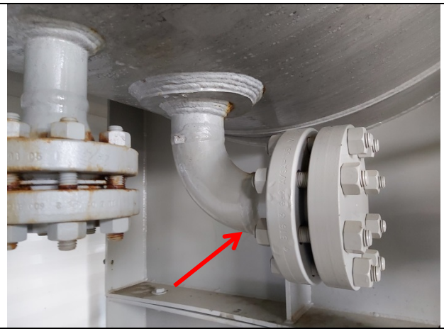
3 in xxs – 9.4/11.8mm isolated pit at DS weld
