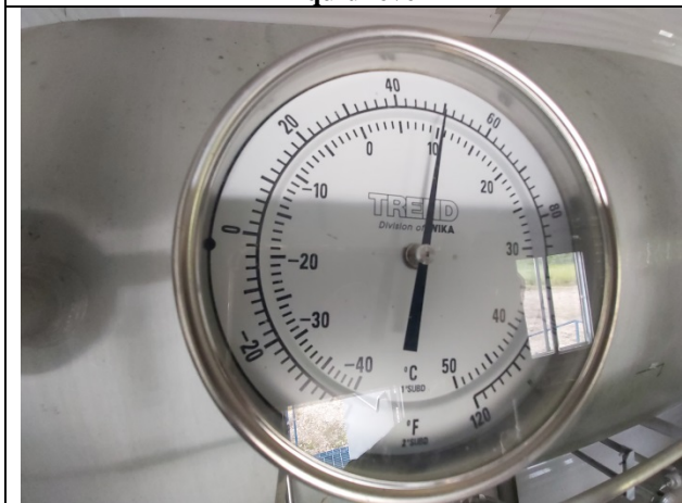
Temperature gauge -40 to 120°F
