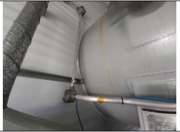
Wall to shell sealed
