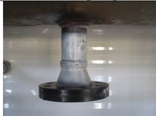
New 2 inch fitting installed
