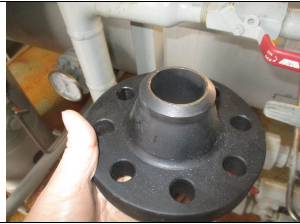
New 2 inch flanged fitting
