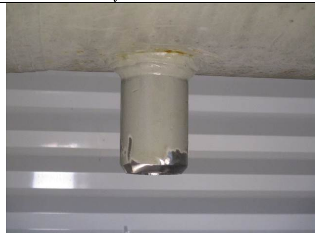
2 inch nozzle prepped for new fitting
