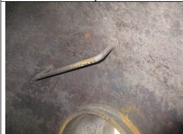
Internal ladder rung
