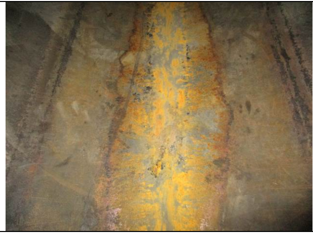
Thin scale on bottom shell – no pitting
