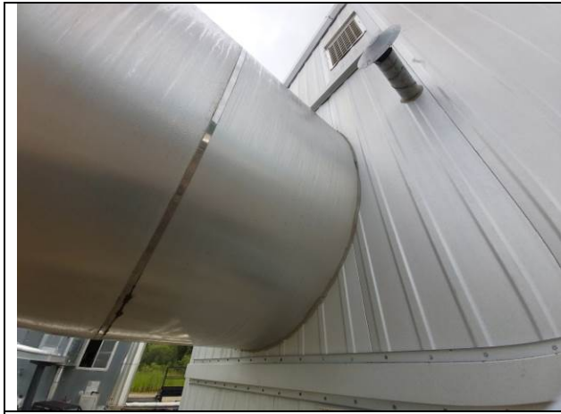
Wall to shell sealed
