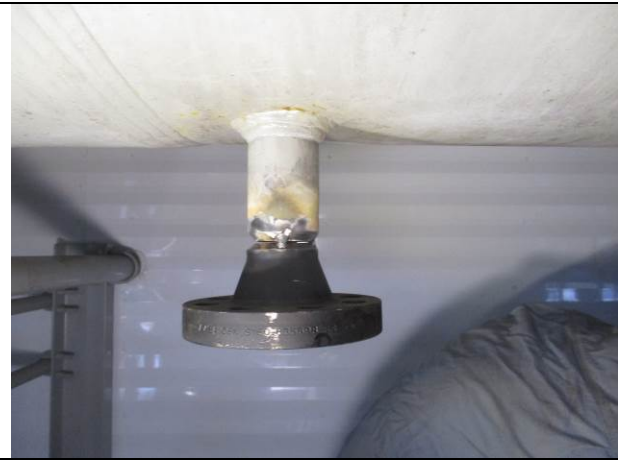
New 2 inch fitting tacked in place
