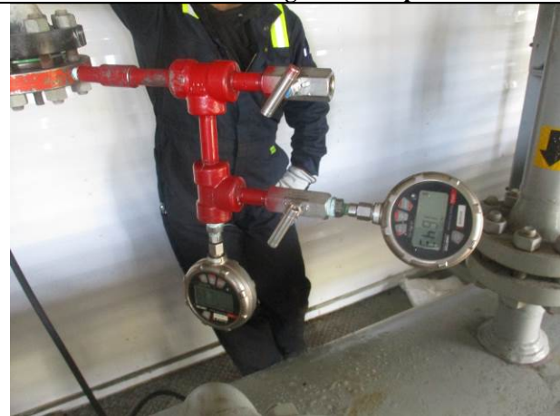
Hydro test set up
