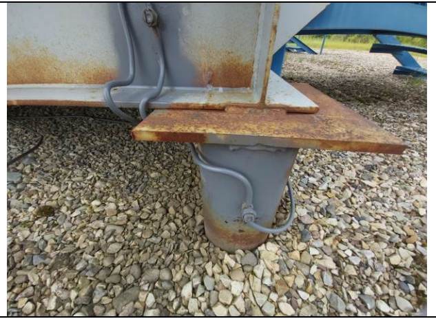
Ground cable attached
