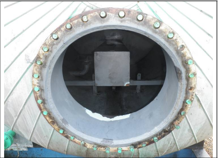
Manway (water dump section)
