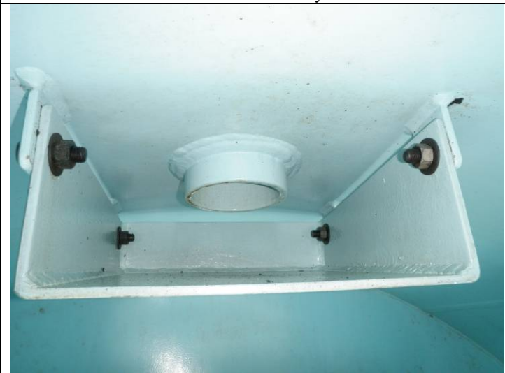
Inlet nozzle and deflector plating (no erosion)
