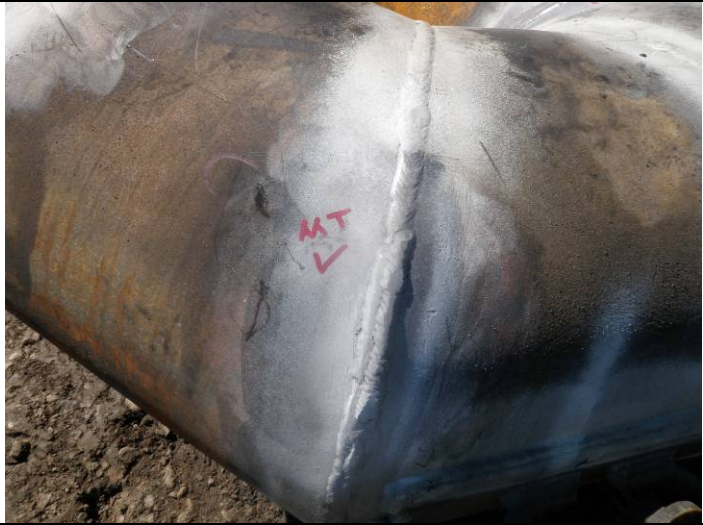
Weld Repair
