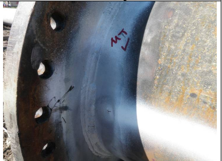
Weld Repair
