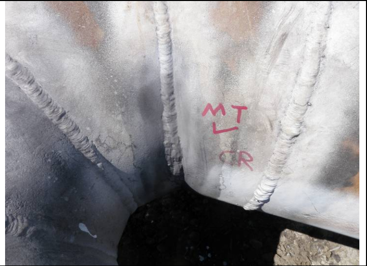
Weld Repair
