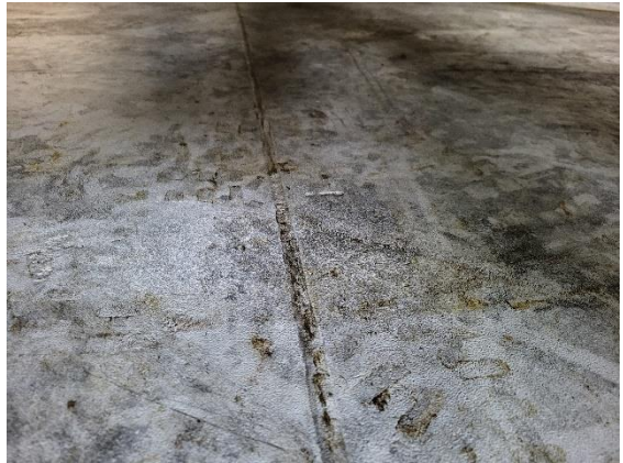
Tank floor weld seam
