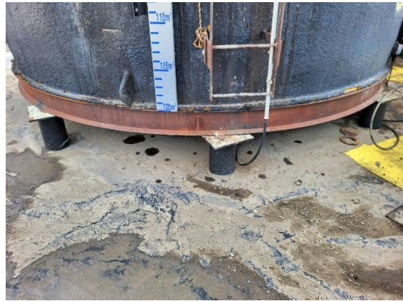
Tank base overview
