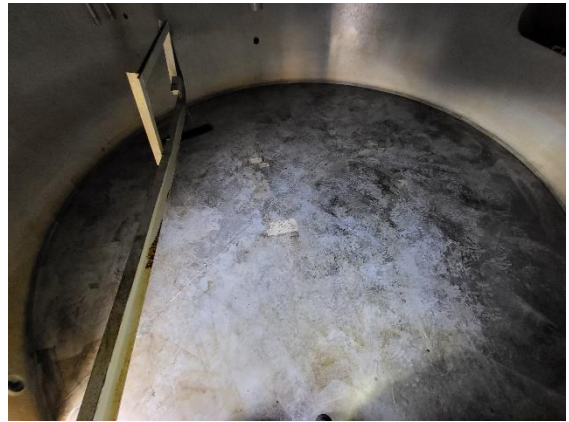
Tank floor overview
