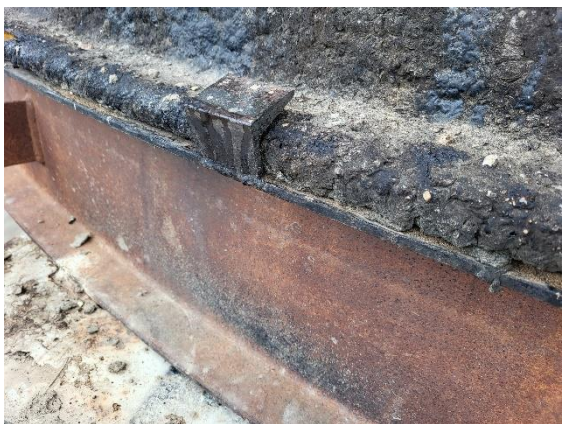
base to skid connection
