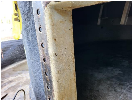
Manway entrance condition
