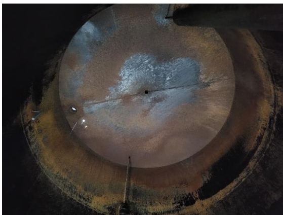
Tank deck overview
