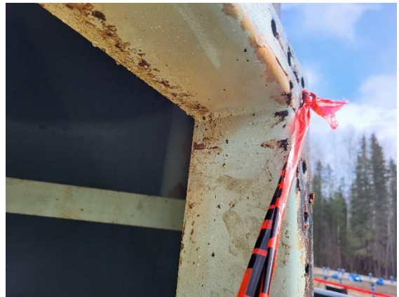
Manway entrance condition
