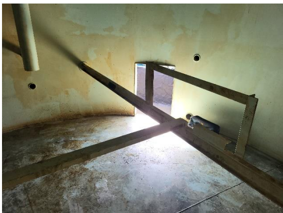
Heating tube support - tube permanently removed
