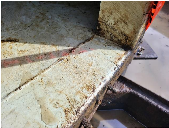
Manway entrance condition
