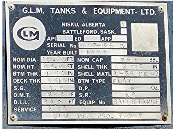
Tank data plate overview
