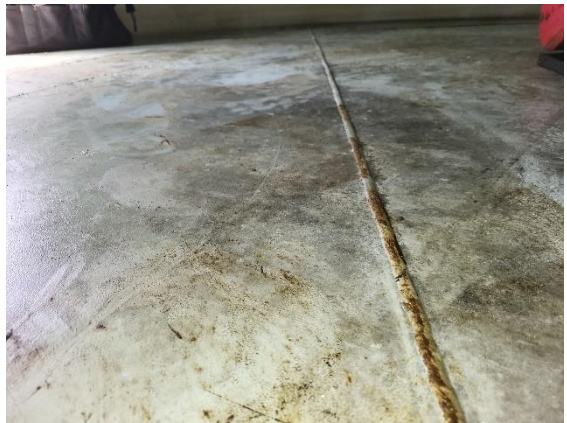
Tank floor weld seam
