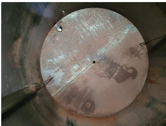
Tank deck overview
