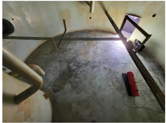
Tank floor overview
