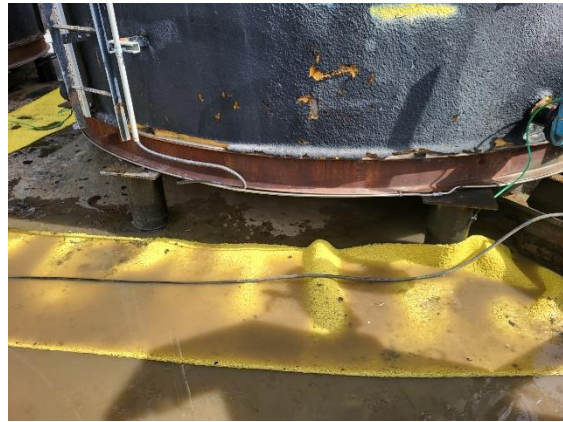
Tank base overview
