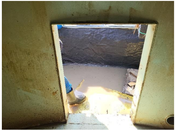
Manway internal overview
