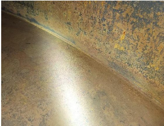
Shell to floor weld seam
