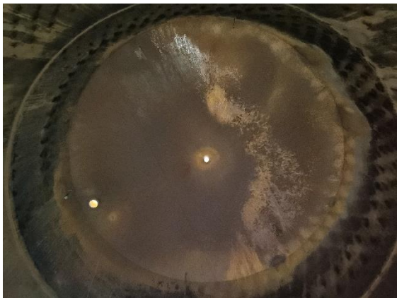
Tank deck overview
