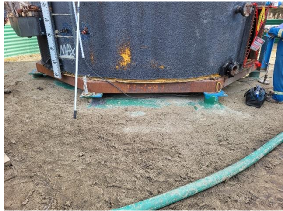
Tank base overview
