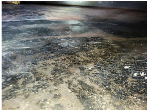
Tank floor overview
