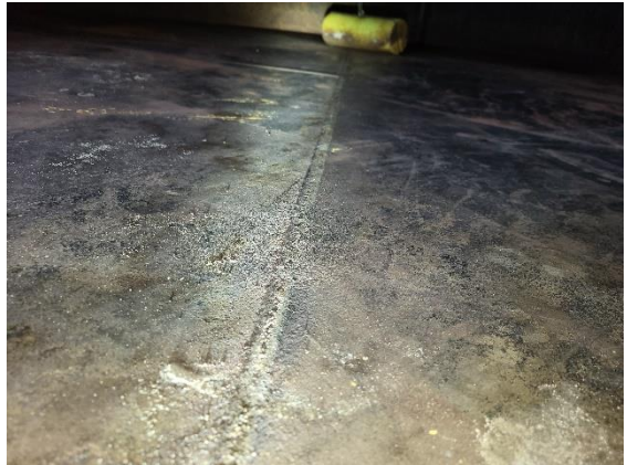
Tank floor weld seam
