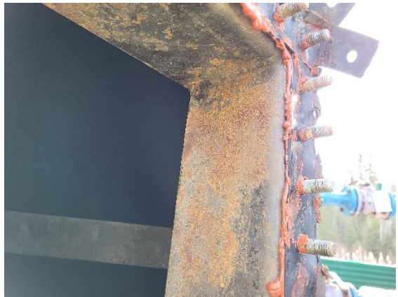
Manway entrance condition
