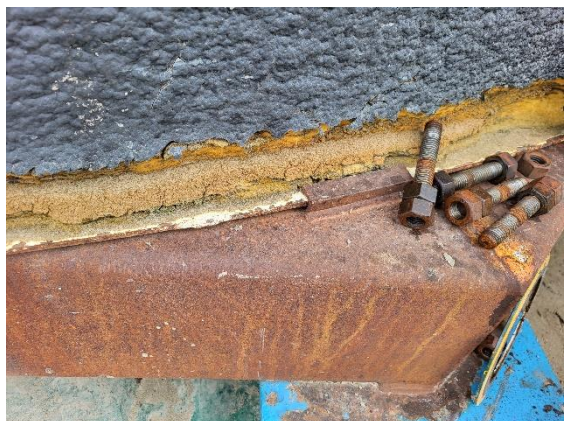
base to skid connection
