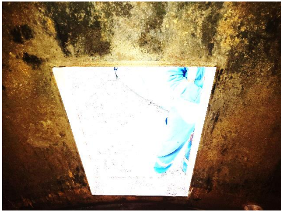
Manway internal overview
