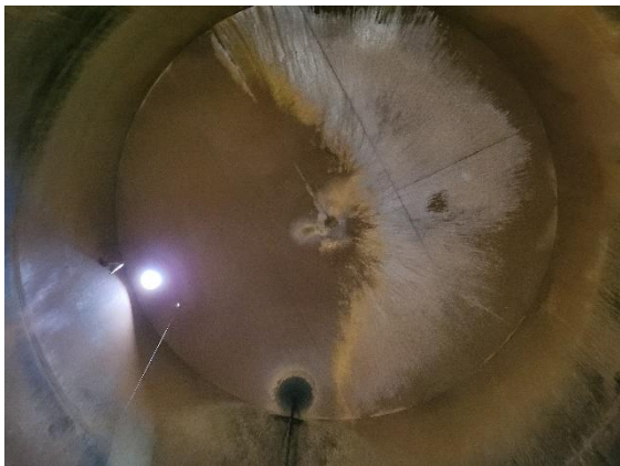
Tank deck overview
