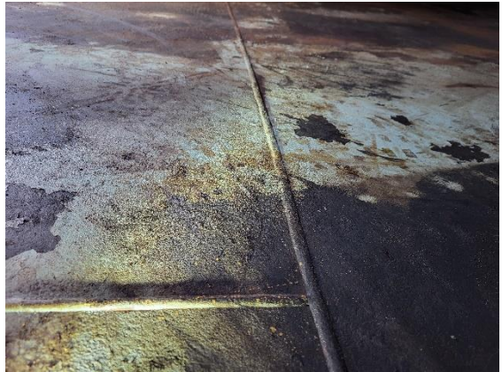
Tank floor weld seam
