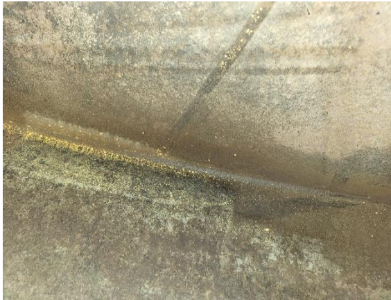
Shell to floor weld seam
