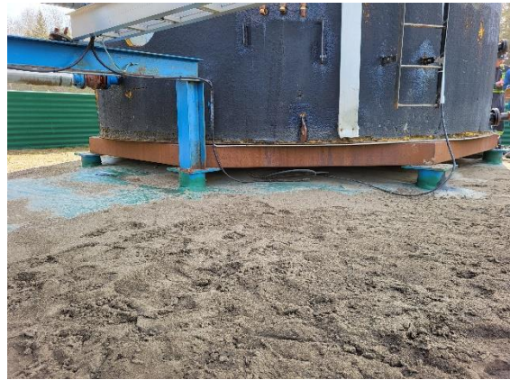
Tank base overview
