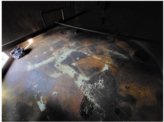
Tank floor overview
