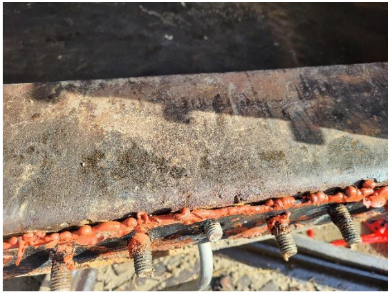
Manway entrance condition
