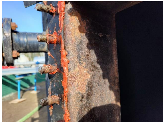
Manway entrance condition
