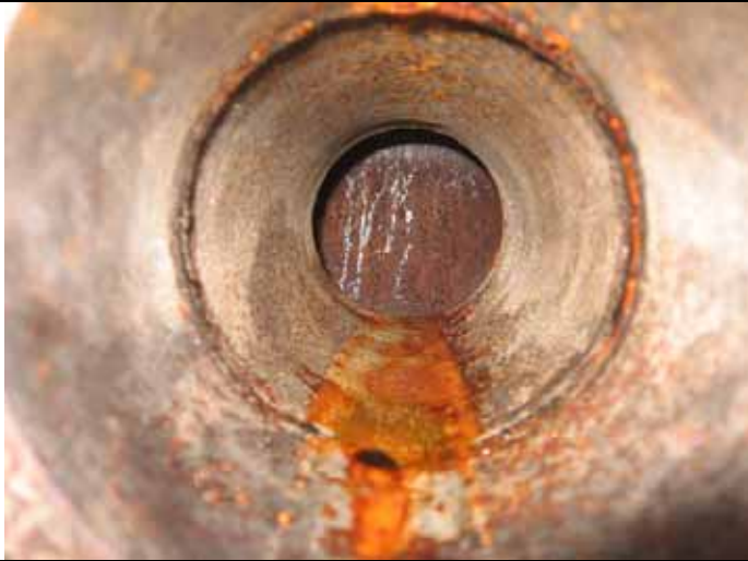
Outlet nozzle with diffuser in place
