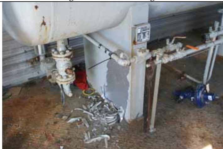
Saddle is in good condition and well supporting
