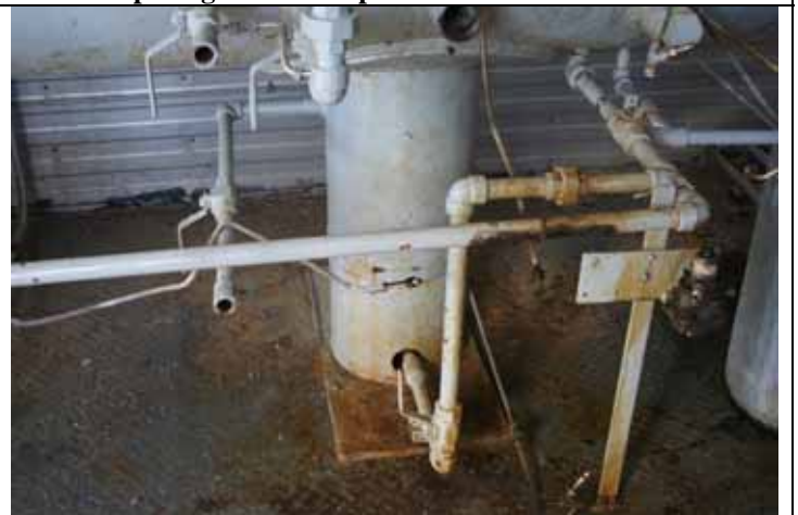
No internal or external corrosion on boot.
