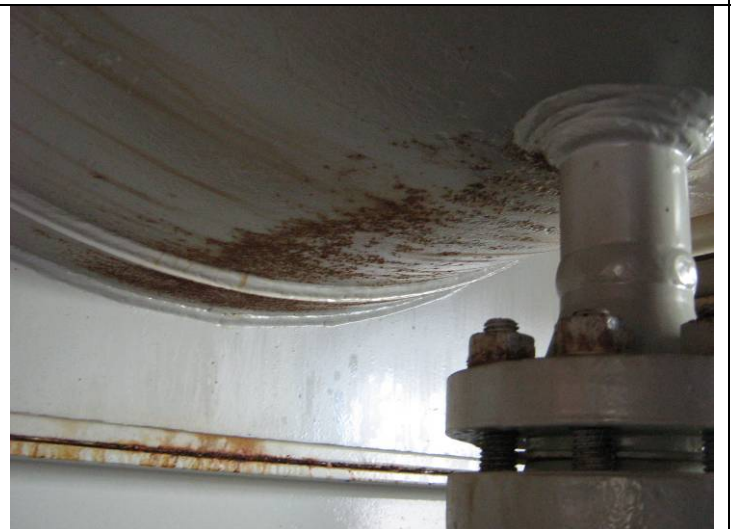
Bottom side nozzle minor rust and scale developing
