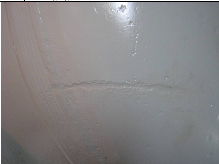
West head pitting coated over (not active)
