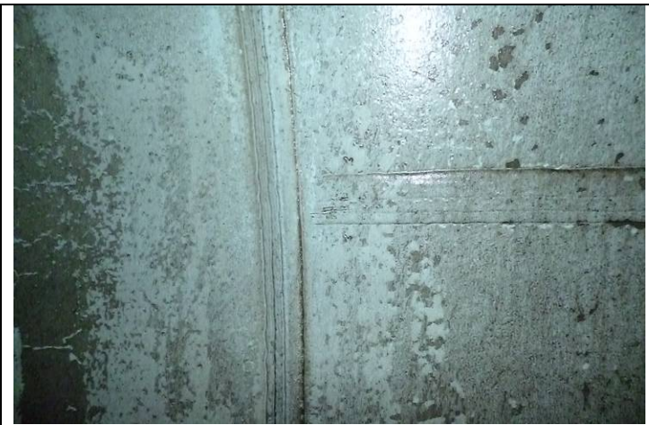
Mid shell tee weld
