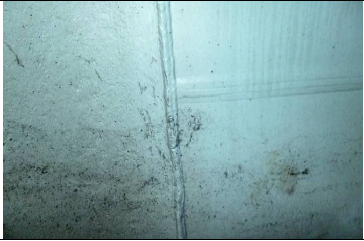
Coated shell tee weld and head weld
