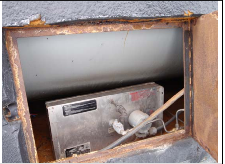
Underbelly paint in good condition
