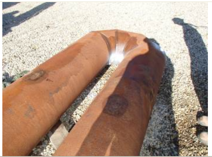
View of the scaling on the fire tube.
