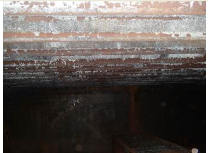
Baffles at the top shell at oil end.
