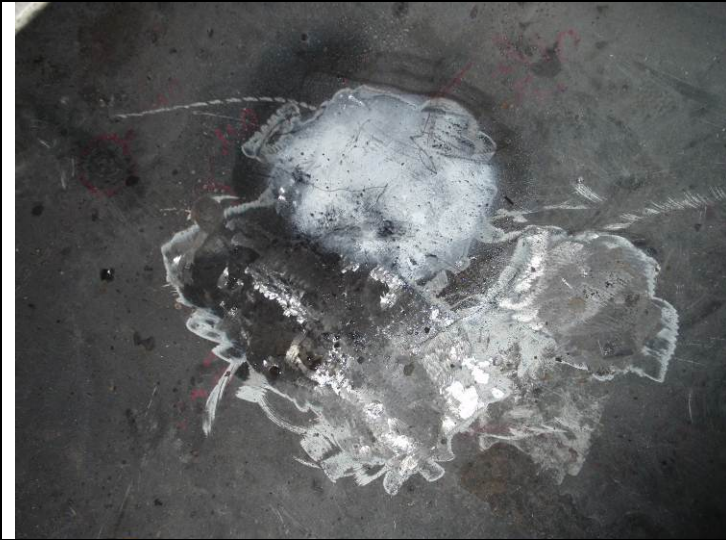
Shell fill welded and ground flush – no indications
