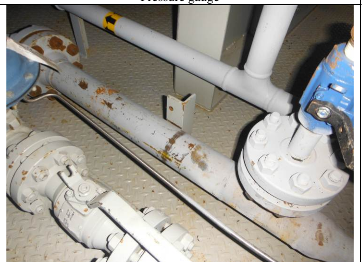
Missing pipe clamp
