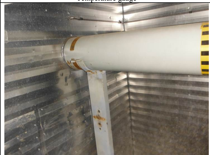
Missing pipe clamp
