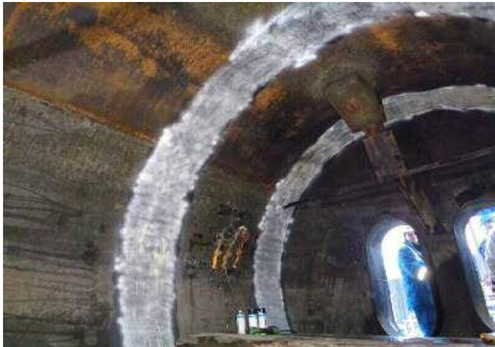
2 x 12" wide bands MPI'd where new inlet horseshoe downcomer is to be welded to shell
