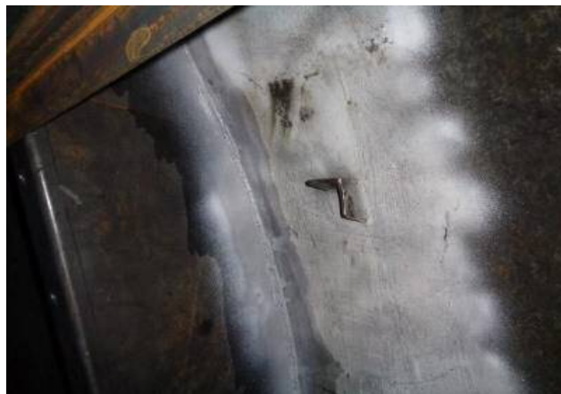
Firetube overhead desand line support beam cut off but not ground flush to shell
