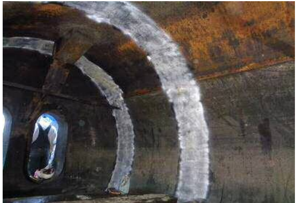
2 x 12" wide bands MPI'd where new inlet horseshoe downcomer is to be welded to shell
