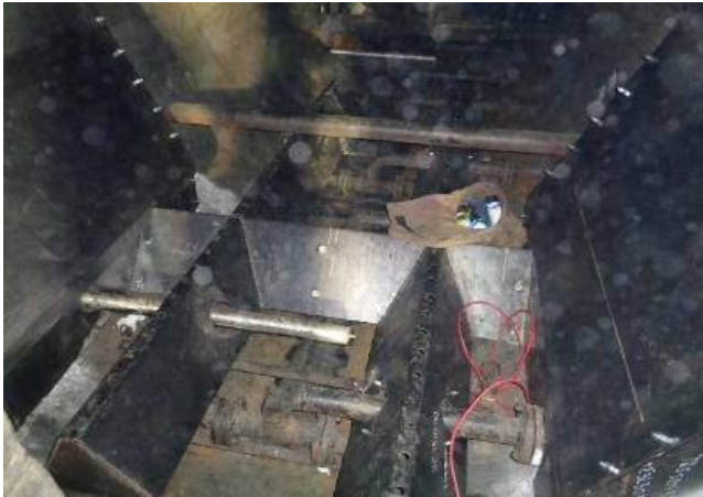
Inlet horseshoe downcomer shroud after all components installed
