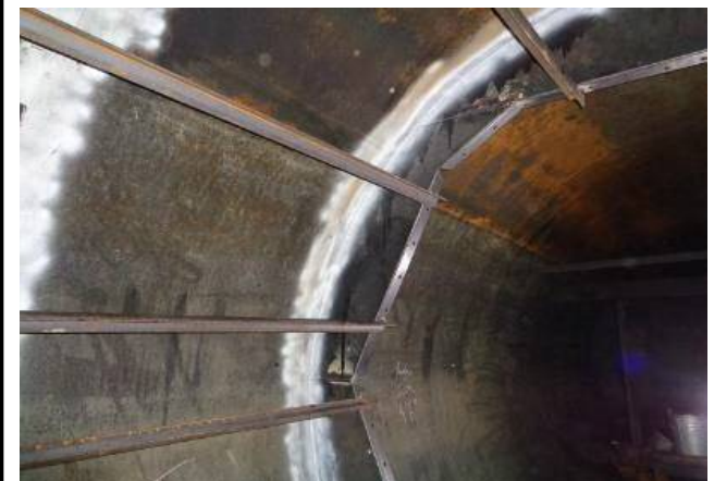
MPI on final inlet horsehoe downcomer to shell fillet welds 12 hours after welding was completed
